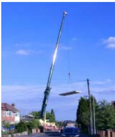
On site a crane is needed to manoeuvre the panels into place and the assembly on site is a job that is best left to specialists, who slot them together and seal the joints. The structure of an average sized house (e.g.150 sqm) can be assembled in two or three days in this way. As well as forming the entire structure of a house, the insulation level of SIPs is so good that they are sometimes used for the infill panels of oak framed houses.
