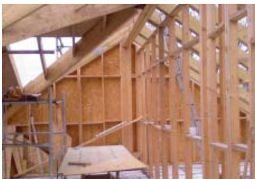
The timber and structure of an open frame are not usually exposed and would not look very attractive even if this were possible. Beyond the breather membrane, the cladding is a matter of choice rather than having to be compatible with the frame. Typical claddings include softwood boarding, tiles, render and a separate masonry leaf. If the latter is used, only an expert eye will be able to spot that there is a timber frame concealed behind it.
