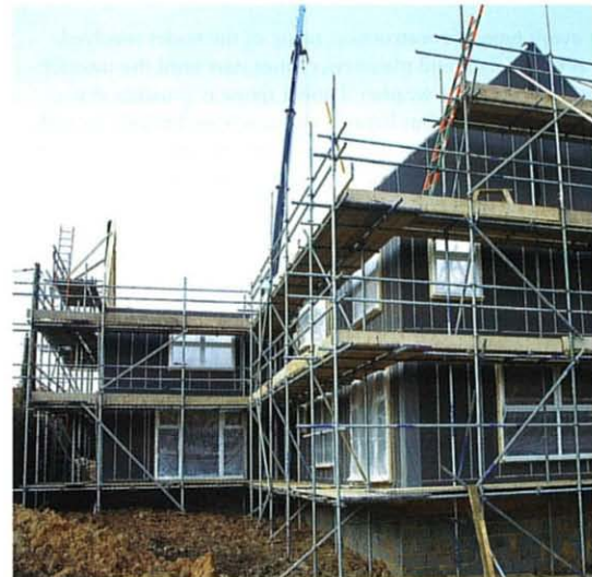
Two storey timber frame under construction
