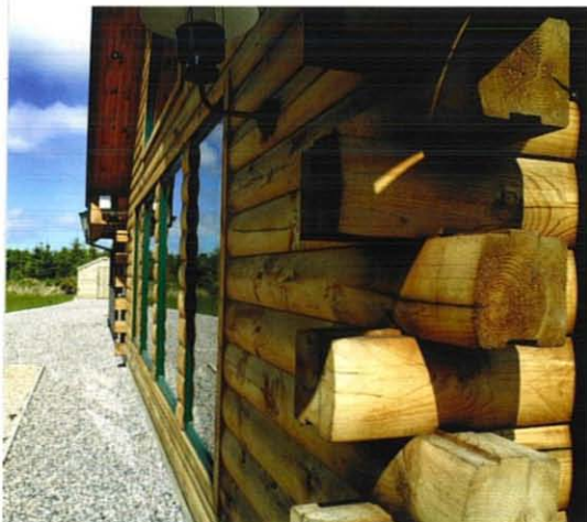
Detail showing thickness of exterior timbers
