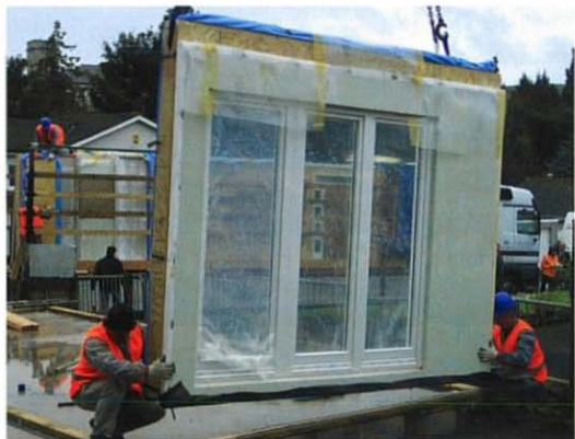
A section of a closed panel house being erected
