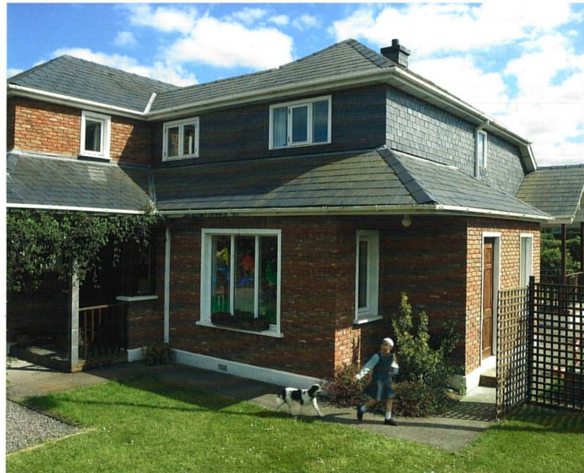
Rear of the same timber frame, house (on previous page)
