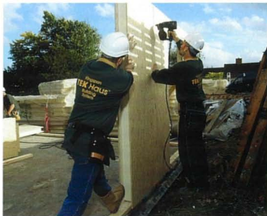
A SIP being fixed in place
