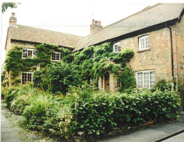
Cottage extension at Tollerton
