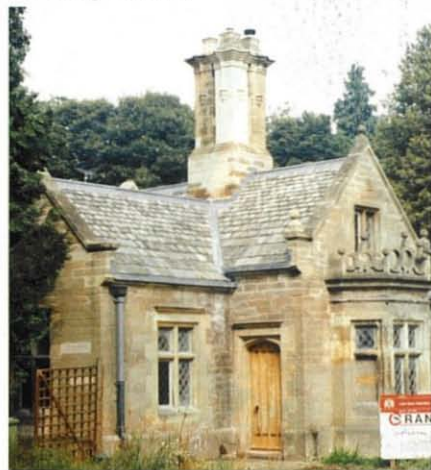
Restoration of Keeper's Cottage, Rufford Park
