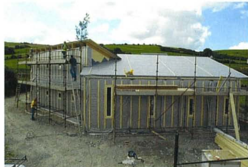
Passive performing house in Clonakilty under construction.
